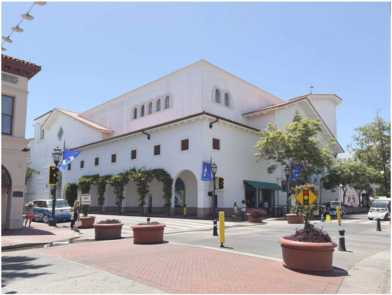
2. STATE ST. & ORTEGA ST. - SOUTH EAST
