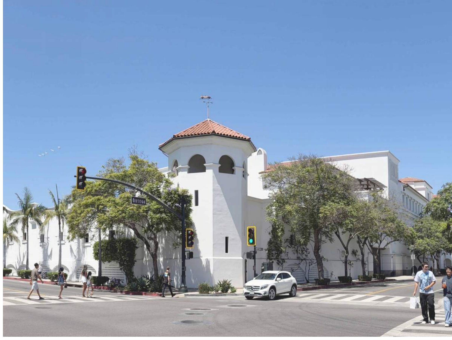
13. CHAPALA ST. & ORTEGA ST. - SOUTH WEST
