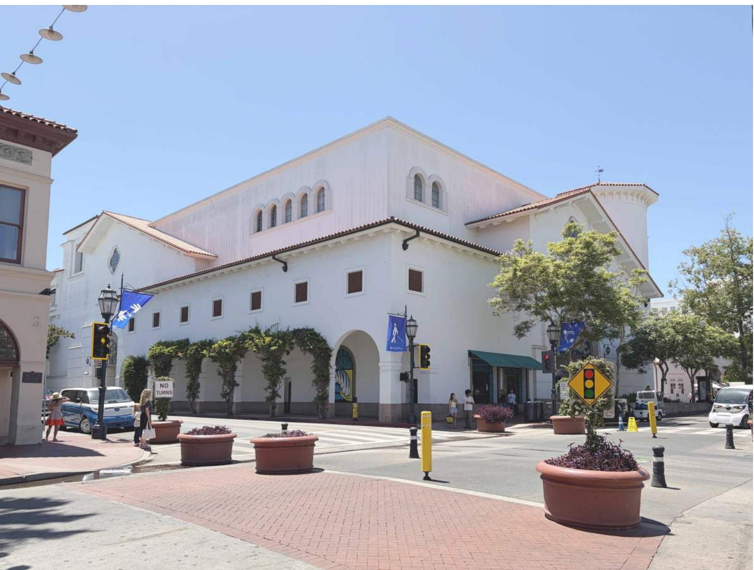
2. STATE ST. & ORTEGA ST. - SOUTH EAST
